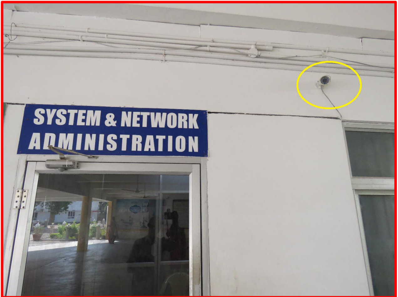
Availability of CCTV at Main Block
